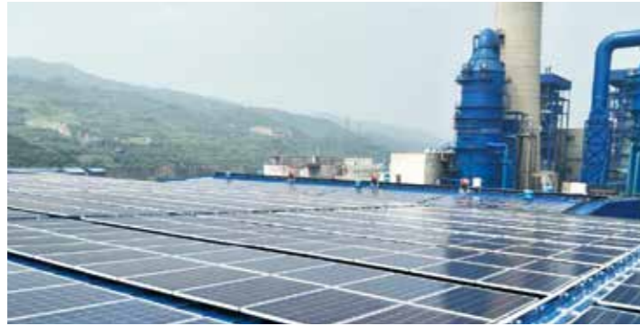
Operation of 50kW String Inverter
