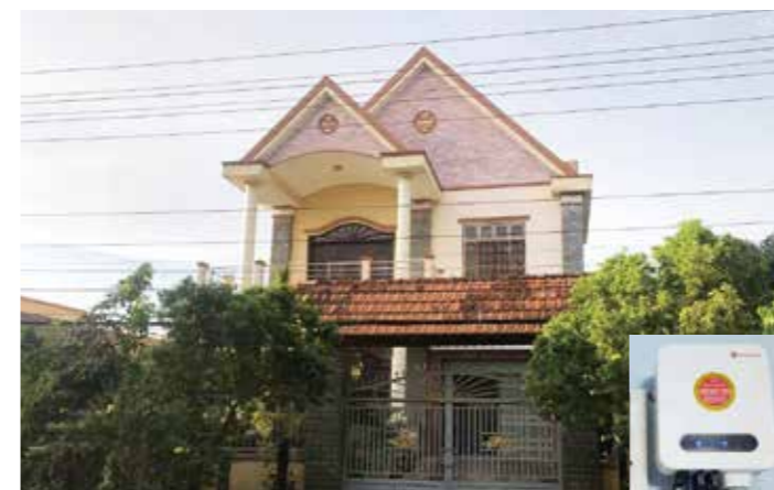
Residential PV Project in Vietnam
